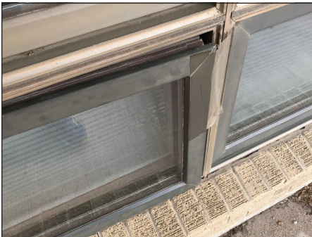
DAMAGED WINDOW
