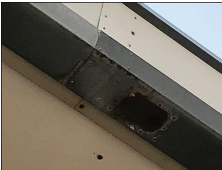
MISSING DOWNSPOUT
