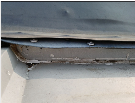
LOOSE ROOF MEMBRANE
