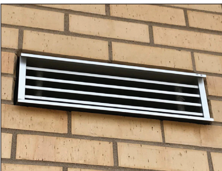
MISSING SEALANT
