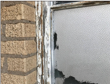
DETERIORATED WINDOW
