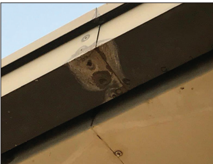
LEAKING GUTTER
