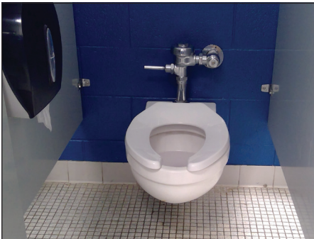
WALL-MOUNTED MANUAL FLUSH VALVE
