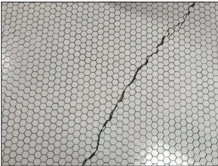
CRACKED FLOORING
