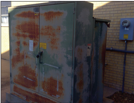
PAD-MOUNTED ELECTRICAL TRANSFORMER
