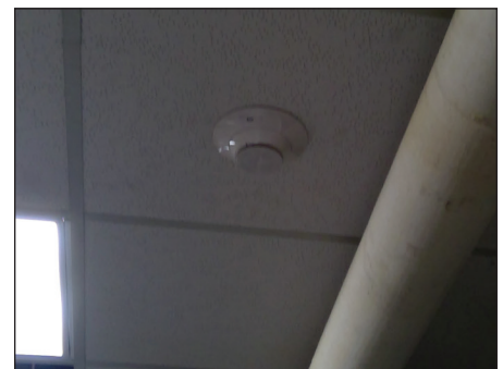
CEILING-MOUNTED SMOKE DETECTORS
