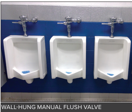
WALL-MOUNTED MANUAL FLUSH VALVE
